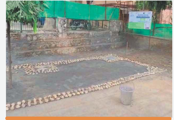
Rain Water Harvesting Structure – B 4 Vasant Kunj
